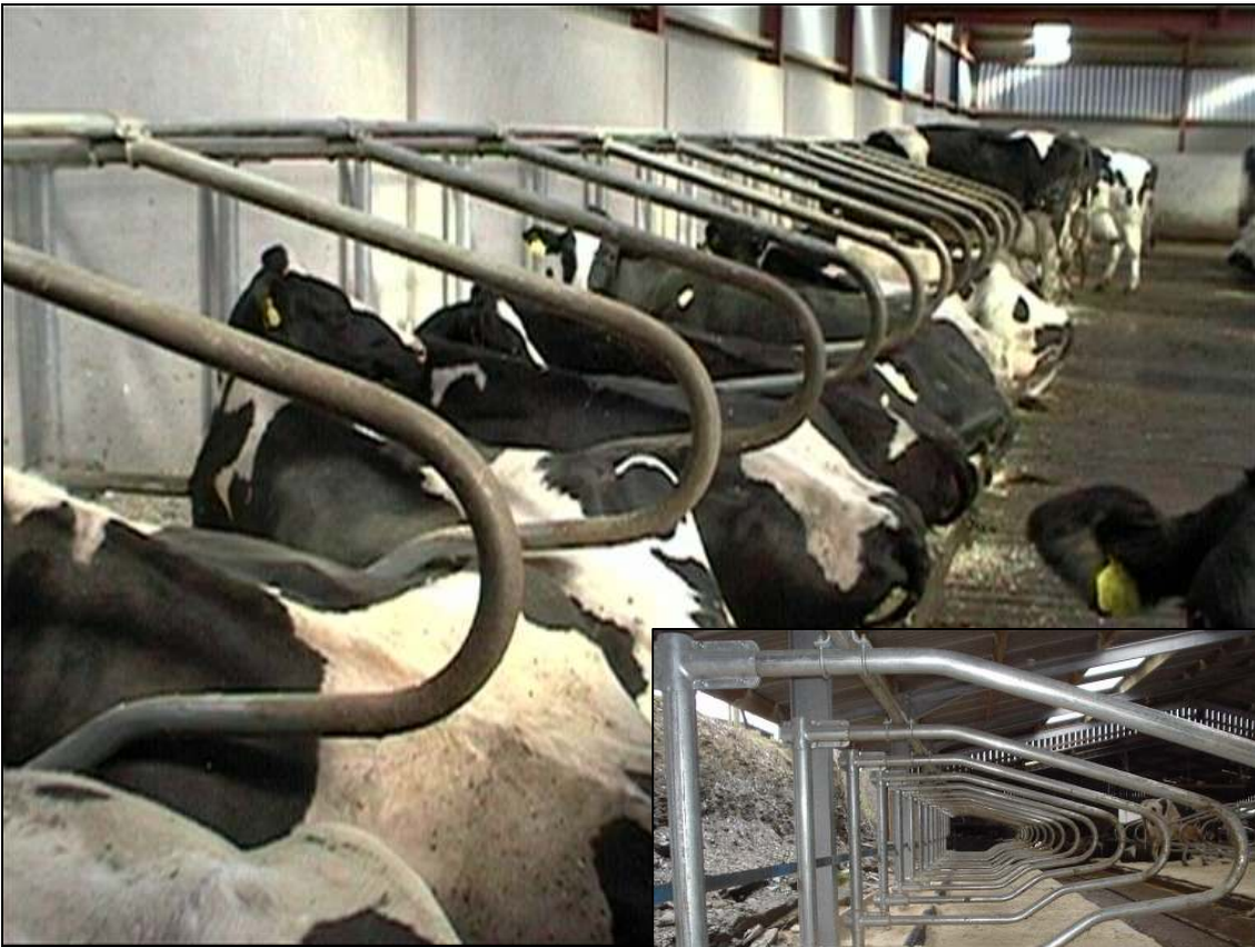
These are 9ft single rows at 3'9" centres. All have 50" high neck rail cubicles.
